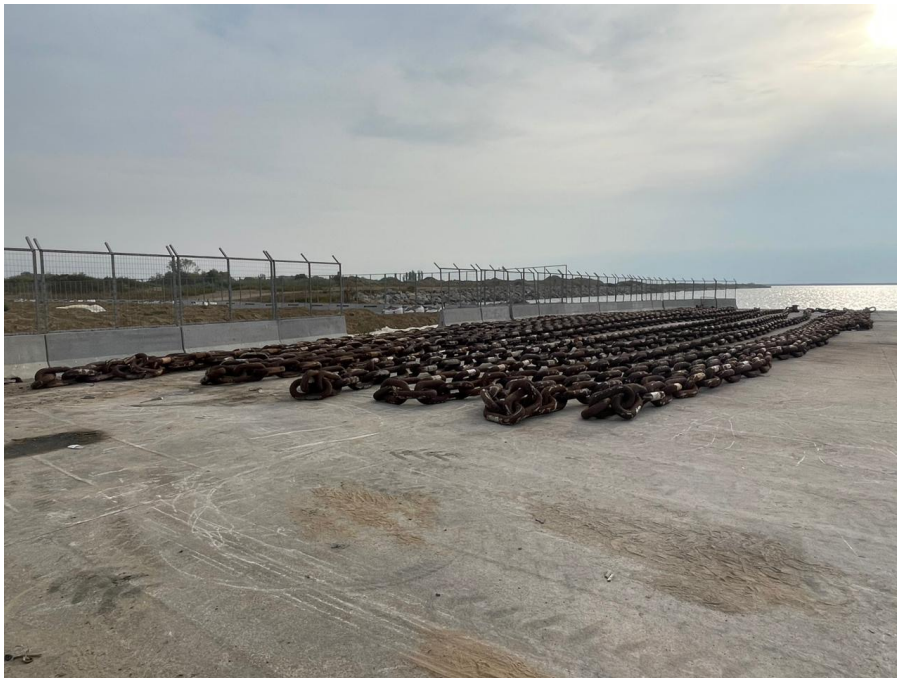
Chains pre-laid to Alexandroupolis Port ready for installation
